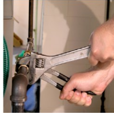
Major Home Repairs
